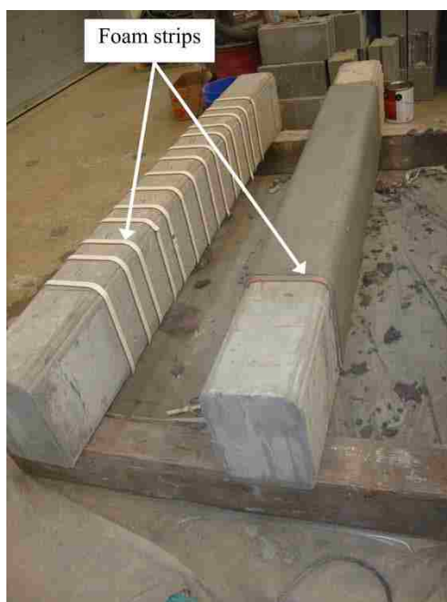
Figure 3. FRCM composite installation.
